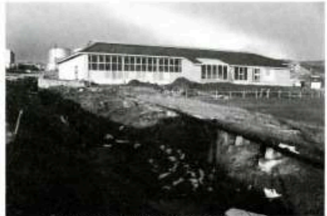
FRONT VIEW OF STANLEY SWIMMING POOL
