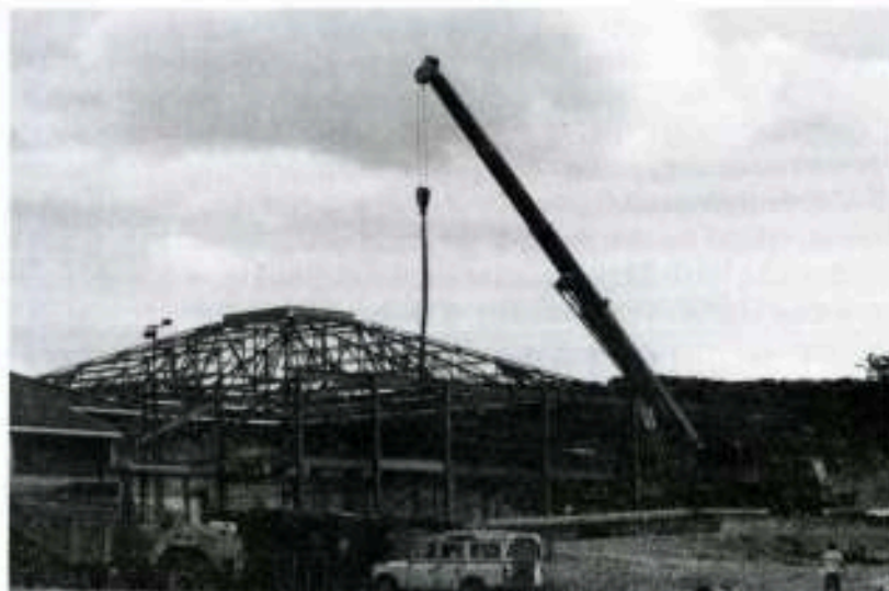
THE NEW STANLEY SCHOOL UNDER CONSTRUCTION (photo: R. N. SPAFFORD)
