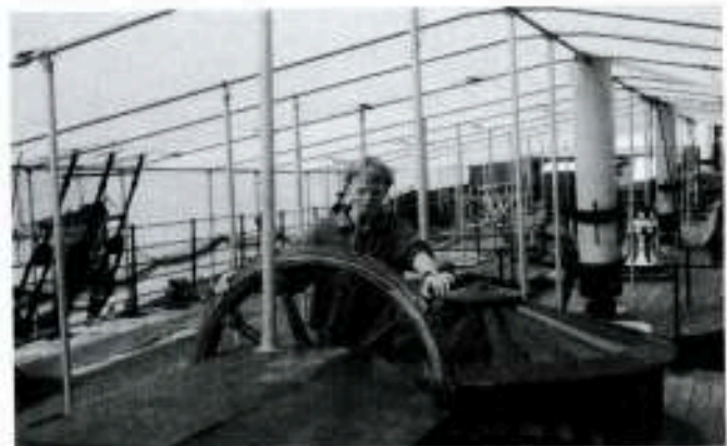
THE TEMPORARY COVER OVER THE WEATHER DECK OF S.S. GREAT BRITAIN
