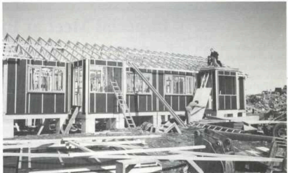
Housing Units Under Construction
